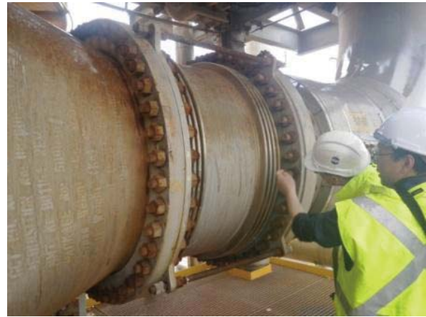
Kurbo's engineers are checking bellows quality of tied universal expansion joint
