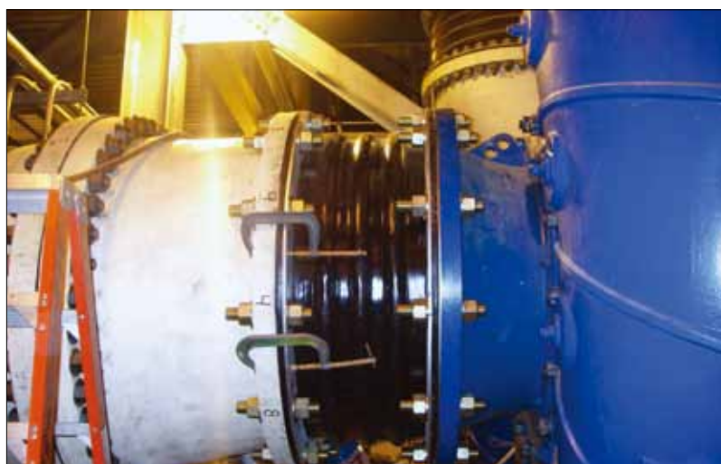
Typical two arch type expansion joint installation for absorption of great movements.
