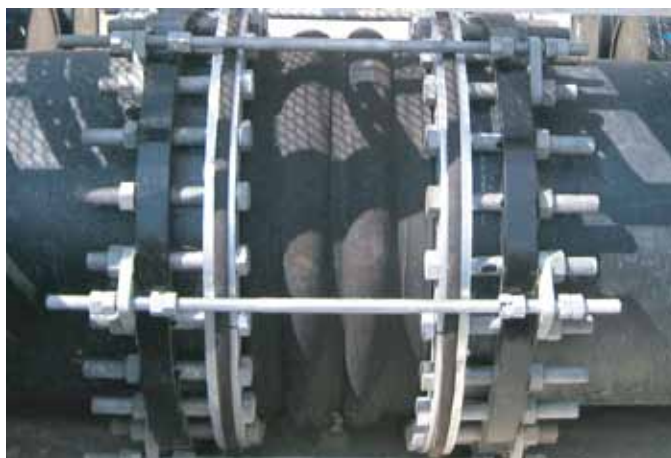
Type 22EP Externally pressurized expansion joint that may be submerged partially when flooded or in monsoon season
