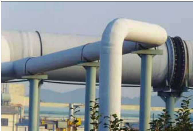
Type 70V –Arch design duct connector in line for odor control in sewage treatment plant
