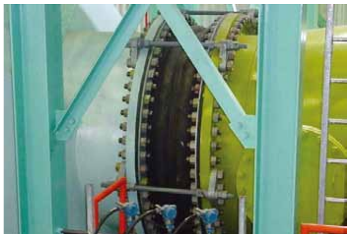
Typical two arch type expansion joint installation for absorption of great movements.
