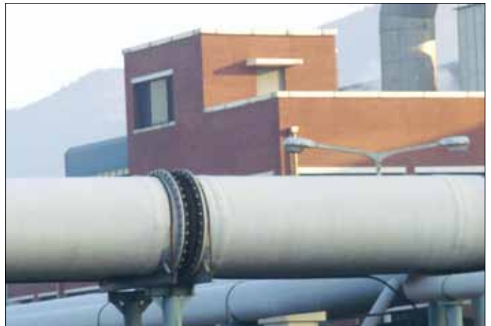
Type 70V –Arch design duct connector in line for odor control in sewage treatment plant
