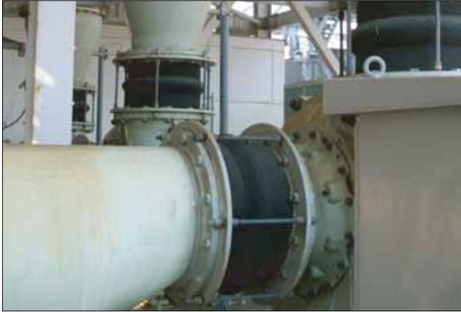
Type 31FF expansion joint with integral flanges
