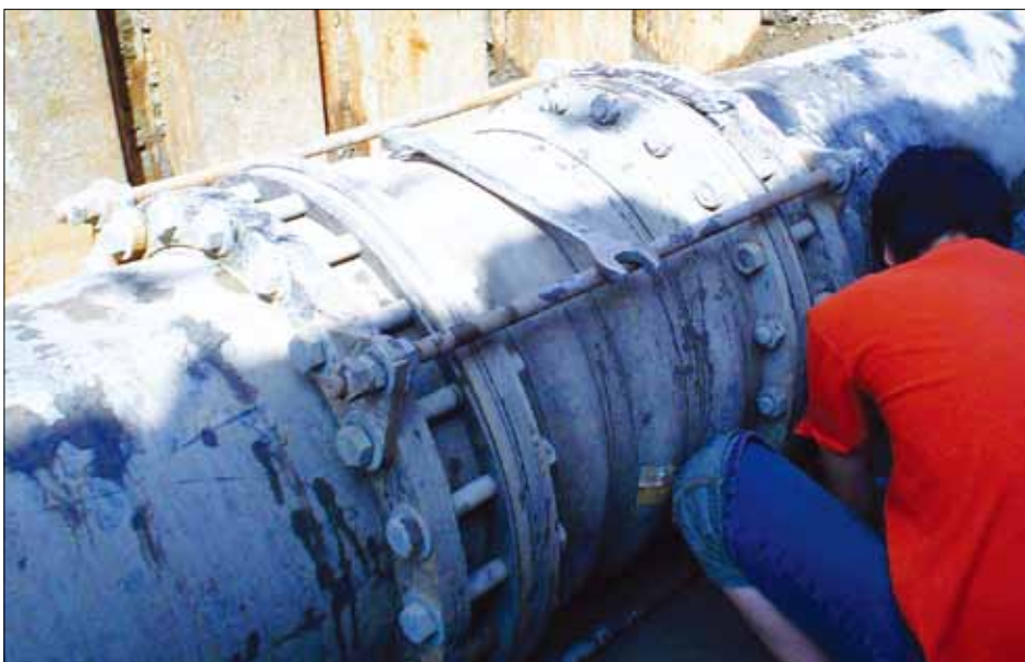
Type 23UG Underground expansion joint for Water distribution and wastewater collection system
